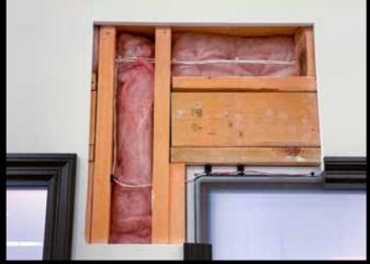
**Step 1** — Terminate wiring to the two conductors at the glass panel or window frame.
