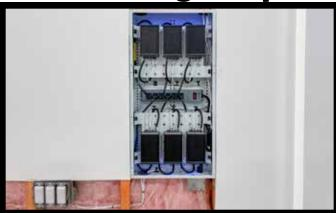
**Step 1** — Find a suitable location for the electronics (i.e. Mechanical Room). Must have a wire path to the window of 100 meters (328 ft) or less, and access to 120VAC.
