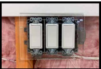
**Step 3** — Run a seperate wire pair to a location in the room for a wall mounted switch or to the automation system if one is being used.
