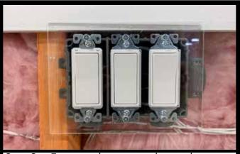
Step 2 — Terminate the wiring at the switching mechanism or the automation system.
