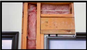
**Step 2** — Run a 18-2 CL3 cable from the electronics location to <u>each glass panel</u>. This will be used to power the windows from Glass Output A and B. **Note** — Leave sufficient wire at the window frame for final connections.
